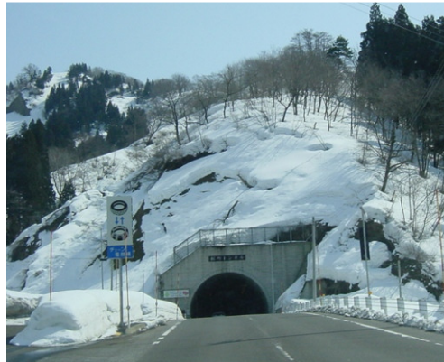
Figura 11 - Efeito “black-hole” à entrada do túnel ( http://www.tanada.gr.jp/picturea/2006-03-05-50tunnel.jpg )
